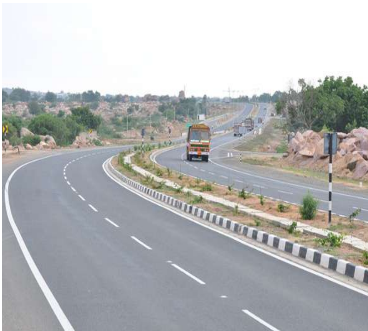
4-LANING OF HUNGUND - HOSPET SECTION OF NH-13 FROM KM.202.000 TO KM.299.000 IN THE STATE OF KARNATAKA UNDER NHDP PHASE-III ON DESIGN, BUILD, FINANCE, OPERATE AND TRANSFER (DBFOT) BASIS (PACKAGE NO.: NHDP-III/NPT/KNT/06)
