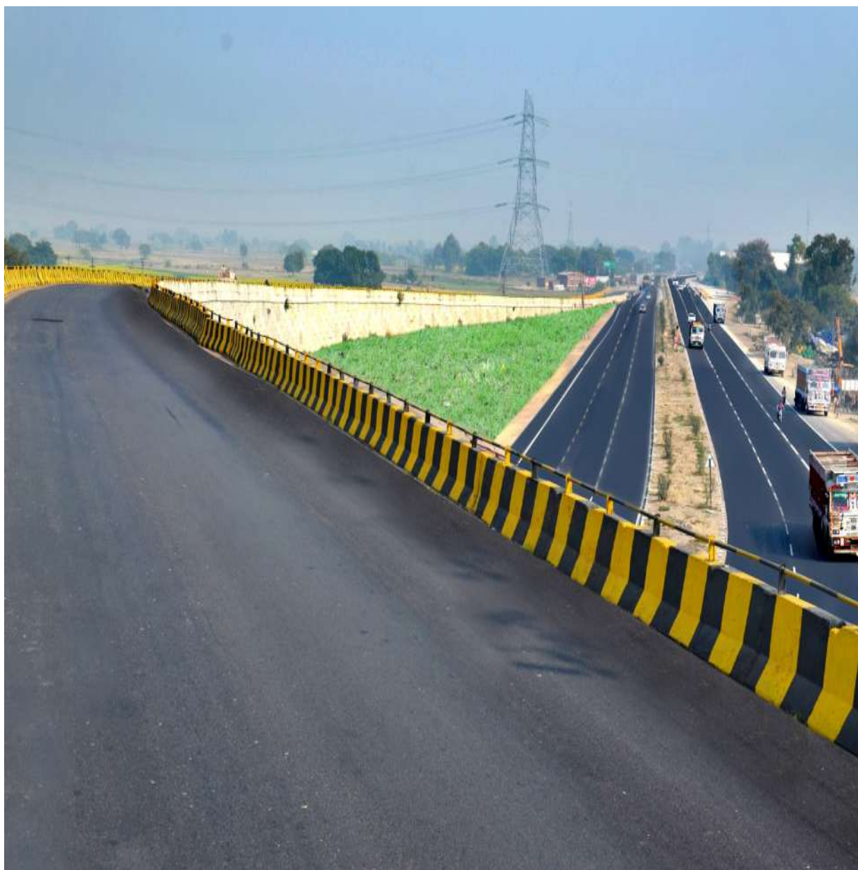
6-LANING OF ETAWAH – CHAKERI (KANPUR) SECTION OF NH-2 FROM KM.323.475 TO KM.483.687 IN THE STATE OF UTTAR PRADESH UNDER NHDP PHASE-V ON DESIGN, BUILD, FINANCE, OPERATE AND TRANSFER TOLL BASIS.
